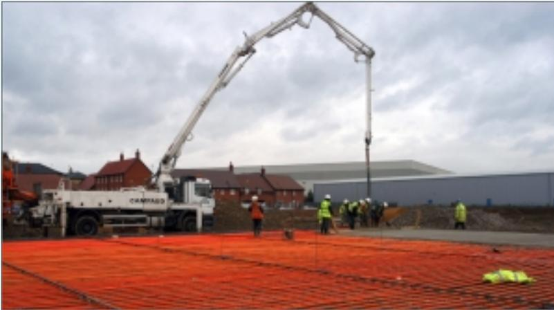
The solar heat collector pipework for the ICAX Interseasonal Heat Transfer system is shown above being installed before the playground is laid. In addition to this system, the wind turbine, solar panels and the TermoDeck building 'mass' ventilation system, the new school features . . .
