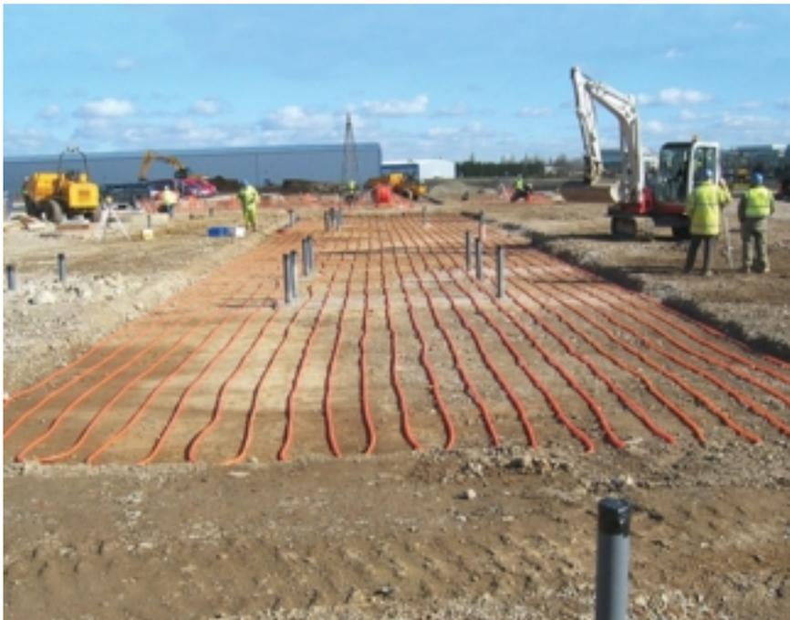
Perhaps the most surprising aspect of the ICAX solution is that the heat vault is simply the earth and rock below the construction being heated. Not only is there no expenditure on a storage medium, but it does not require a special retaining tank or insulating wall to contain it.
