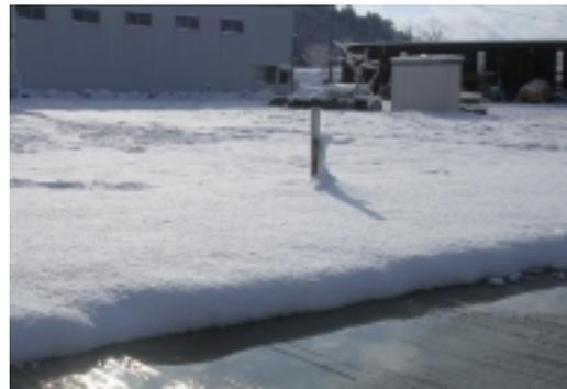
The ICAX technology has been licensed by Misawa in Japan for this experimental site at Hiroshima, where the area to the front of the picture is being kept free from ice and snow using heat captured during the Summer.
