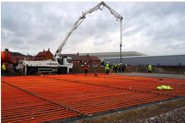
Solar collector construction
