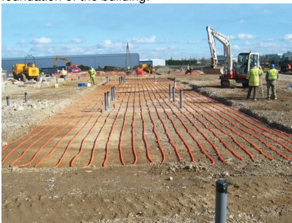
ThermalBank installation at Howe Dell
