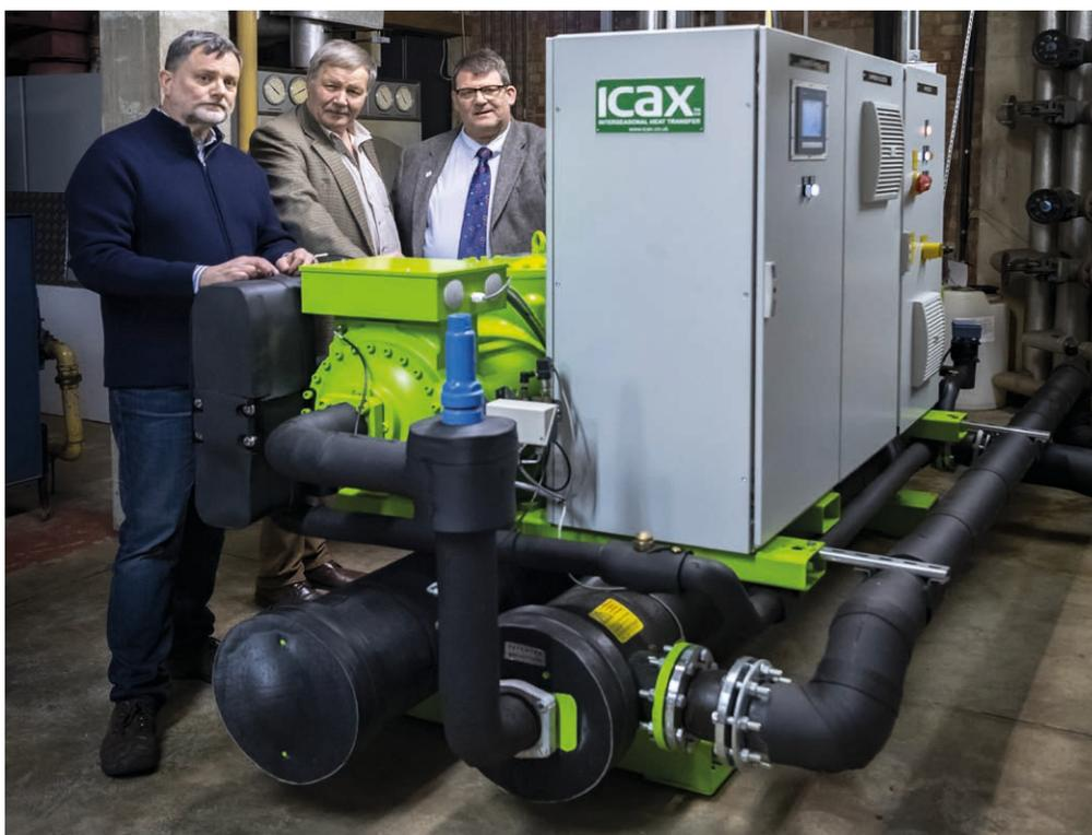
A modern, high temperature heat pump – this has been directly substituted for gas boilers in a plant room, avoiding the need to refurbish heat distribution systems
